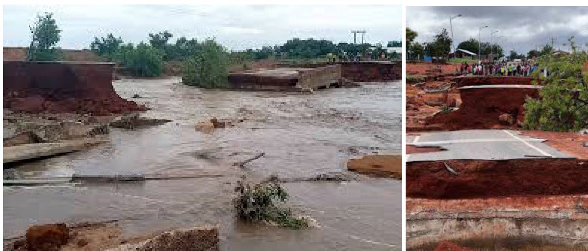
Figure 12: Flood cuts off highway from Walewale to Nalerigu
