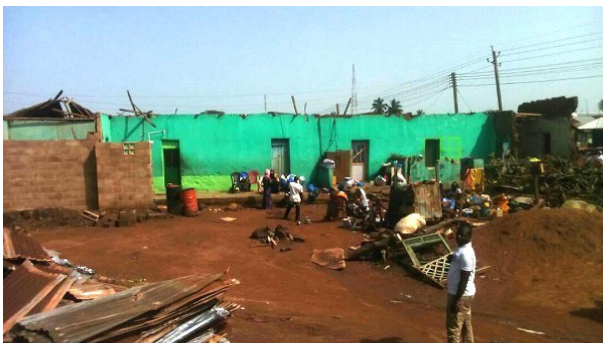
Figure 8: A heavy downpour of rain coupled with strong winds rendered some residents homeless in Wenchi in October 2017
