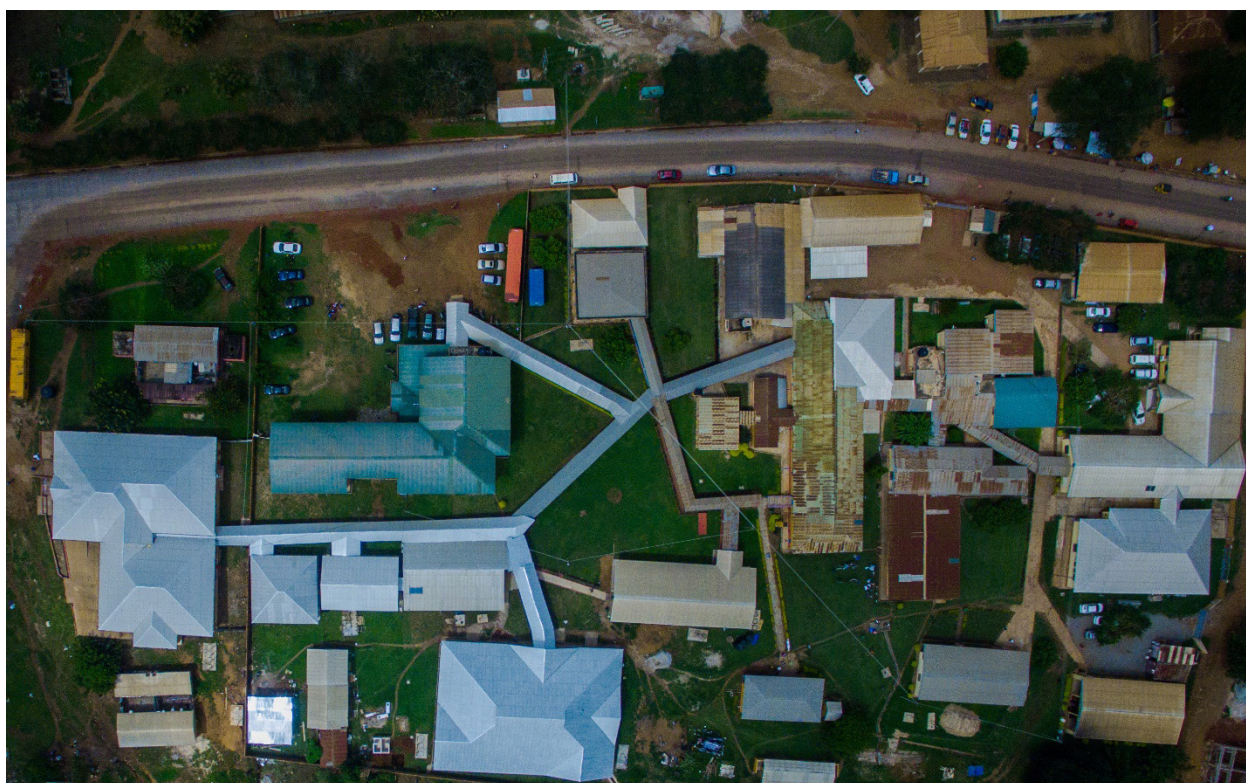
Figure 4: Aerial overview of the Wenchi Municipal
